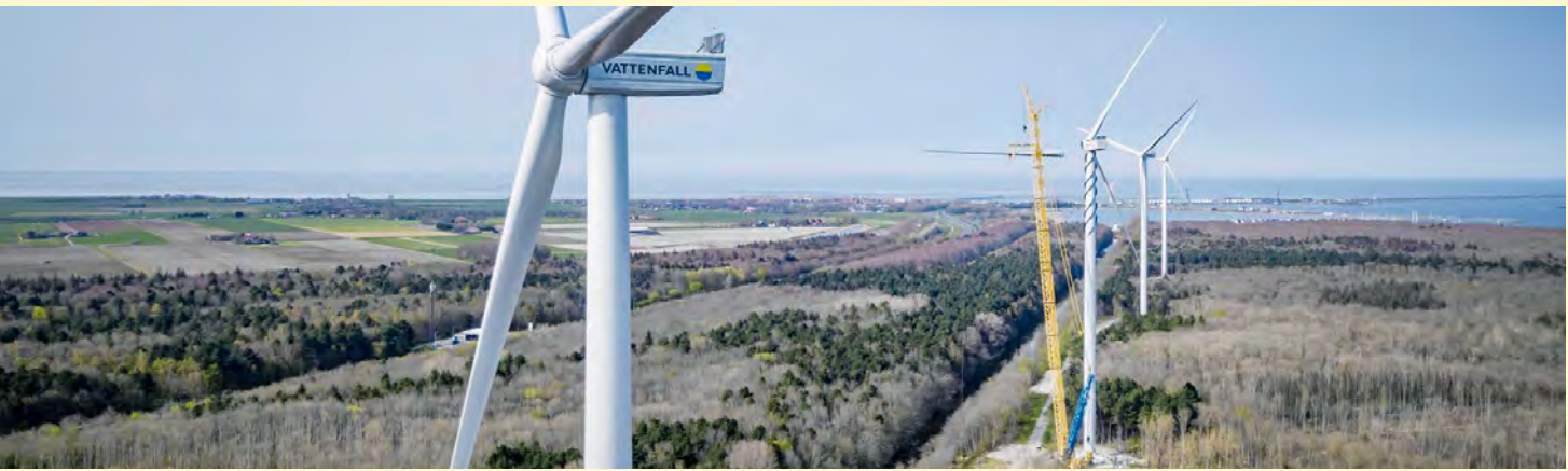
Princess Ariane onshore wind farm in the Netherlands.
