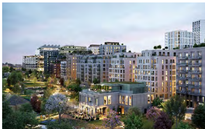
London Brent Cross South - Vattenfall's first district heating network in the UK.
