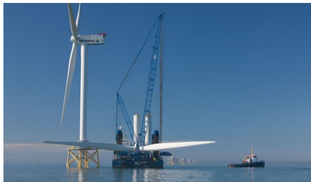
Installation of wind turbine at Ormonde offshore wind farm, UK
