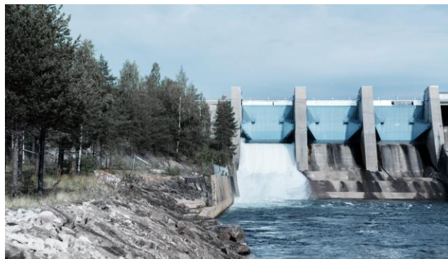
Laxede power plant, Sweden
