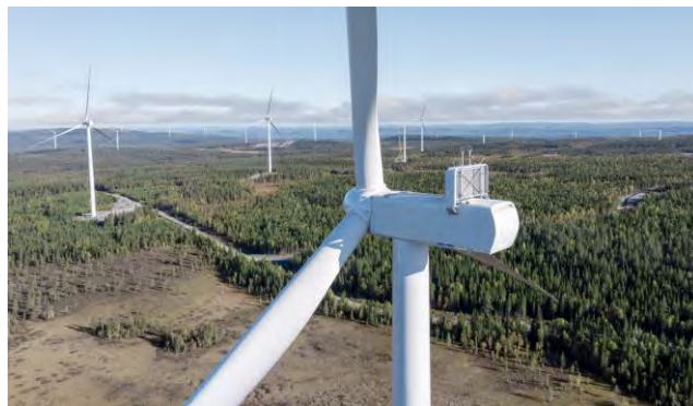
Blakliden Fäbodberget, Scandinavia's largest onshore wind farm to date
