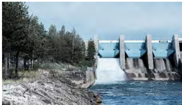
Laxede power plant, Sweden
