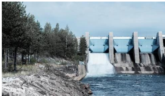
Laxede power plant, Sweden
